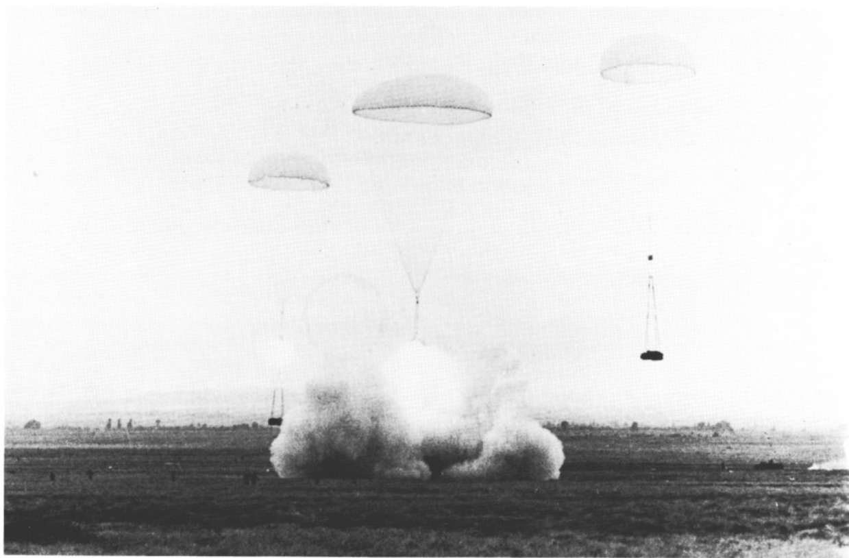
The Soviets have pioneered the use of heavy platforms for airborne landings; these appear to be BMD platforms. Posts protrude beneath the platforms, triggering a retro-rocket to soften the impact of the main structure.
